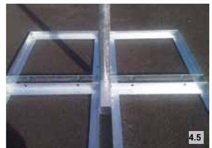
by the M10 nut and tighten until there is no movement between the T-bar and the base tray.
