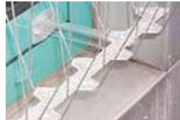
3.10 Spikes can be easily fitted to casement windows where there is a need to protect the window ledge from perching birds but maintain the use of the window for ventilation. This is achieved using our specialist Polycarbonate Window Clips (BS359) which snap-on to the polycarbonate base of the spike strips. Use two window clips per 33cm section of spike. Attach one clip to either end of the spike strip.
